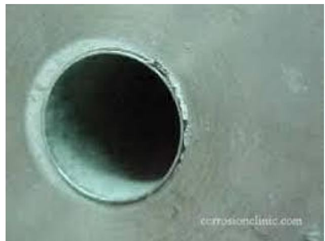
Figure 8: Instance of crevice corrosion (corrosionclinic.com)
