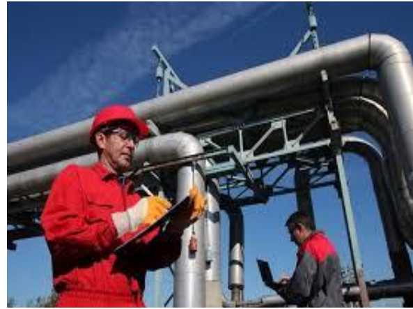
Figure 13: corrosion control and painting and monitoring (capex.com.ng and corrosionpedia.com).
