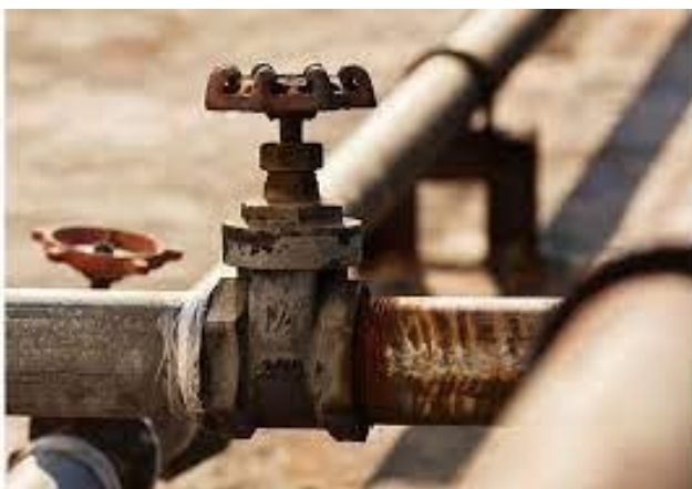
Figure 7: Instance of Galvanic Corrosion (corrosionpedia.com)
