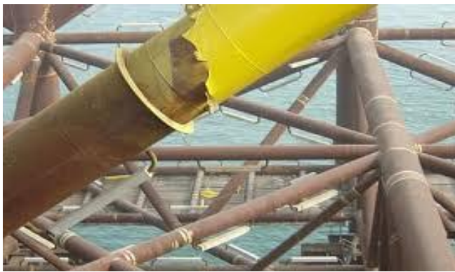
Figure 6: Instance of Oxygen Corrosion (ipdlabservices.co.uk).
