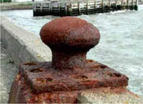
Figure 2: Instance of general or uniform corrosion (nace.org)
